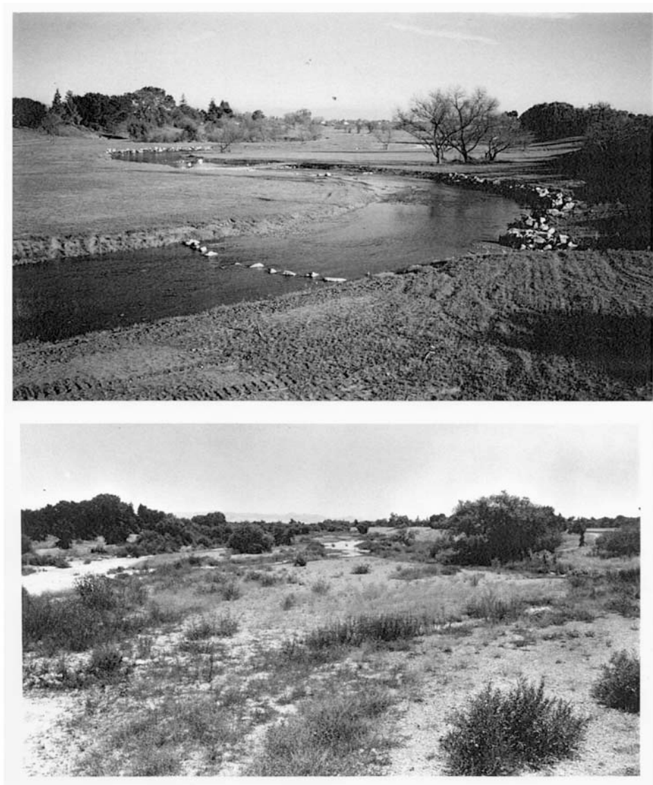
Figure 2. Photographs looking downstream along the channel of Uvas Creek in coastal California. (a) In January 1996, approximately 2 months after construction of a channel reconstruction project that emplaced a meandering channel form, and (b) in June 1997, after the project was destroyed during storm flows with a return period of 5–6 years. Historical geomorphological analysis indicated that the channel reach had been braided historically, typical of streams draining the Franciscan Formation in the California Coast Ranges, with episodic flows and high sand and gravel transport. (After Kondolf et al. [2001, Figure 5] with kind permission of Springer Science and Business Media.)
